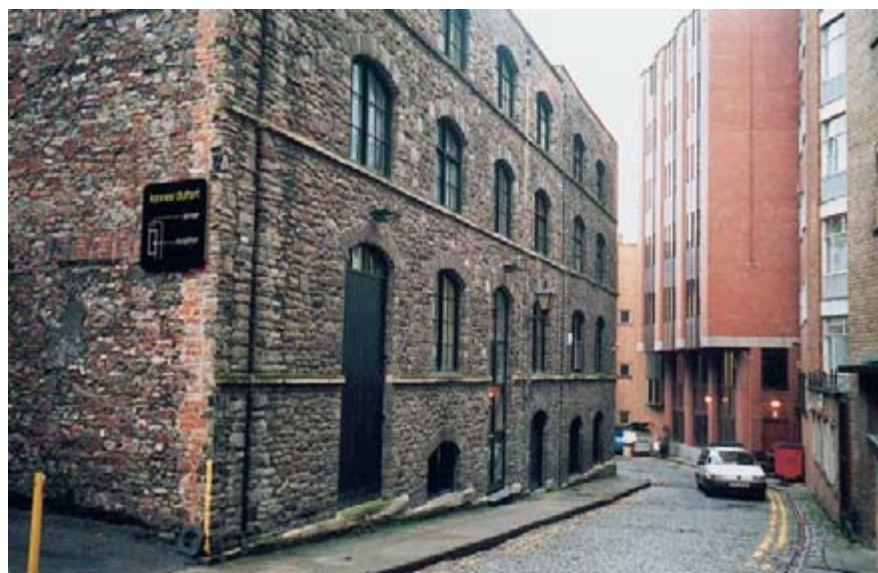
The exterior of the building
