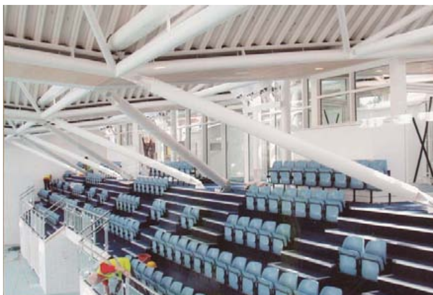
View of roof at seating level
