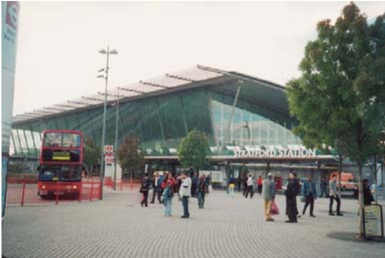
Exterior view to entrance
