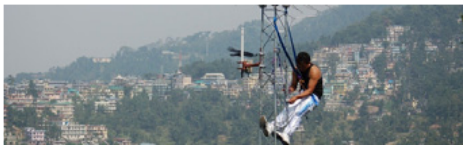
Figure 11.5: Dharamsala installer working on a tower
