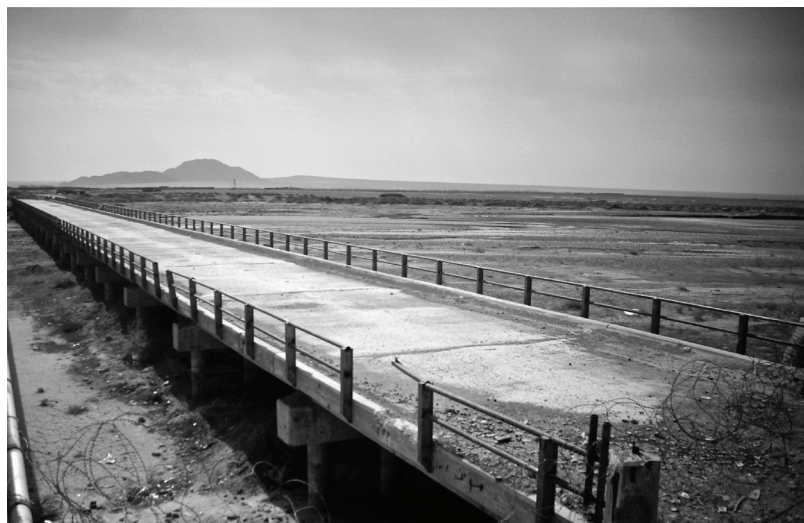
Arghestan Bridge, Kandahar province
